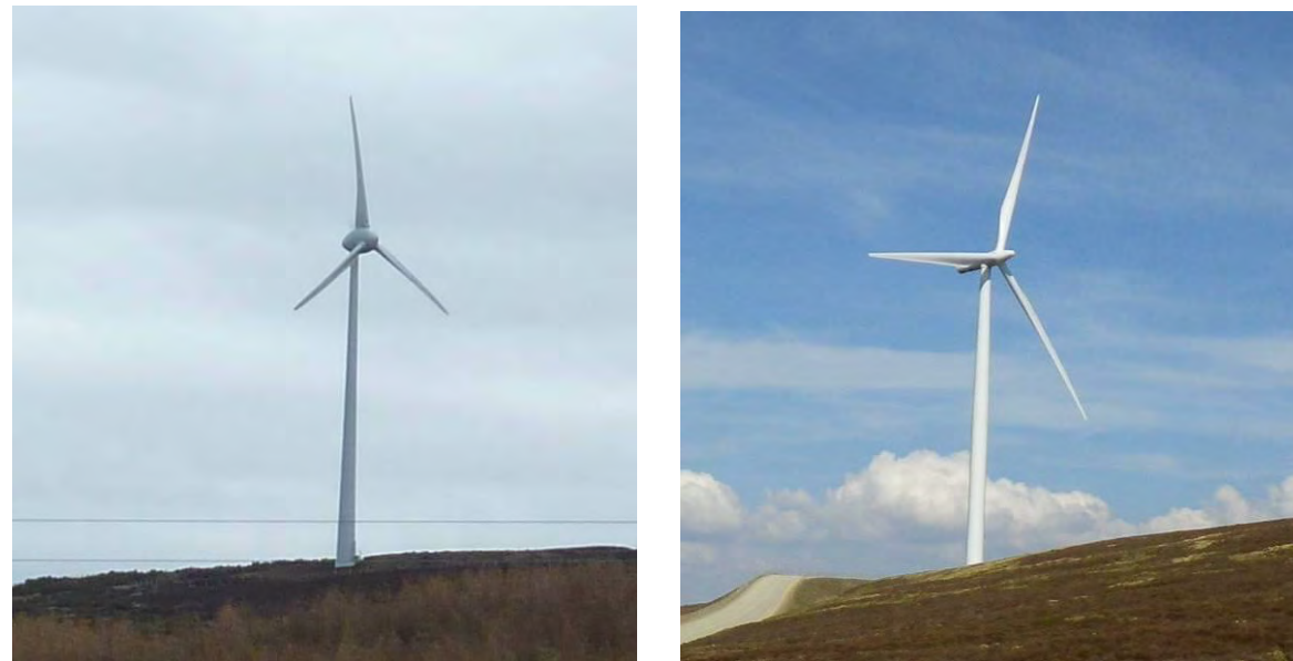
Enercon and Siemens turbines have different nacelles, blades and towers leading to significant differences in appearance
